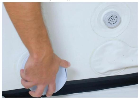
Reason 4: The inlet and outlet of the pump are blocked by scale. Solution 4: Cut off the power then remove the pump. After that clean the scale on the in/outlet ports.
